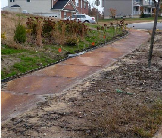
*Acid Sulfate Soils can stain and degrade concrete and other surfaces*
